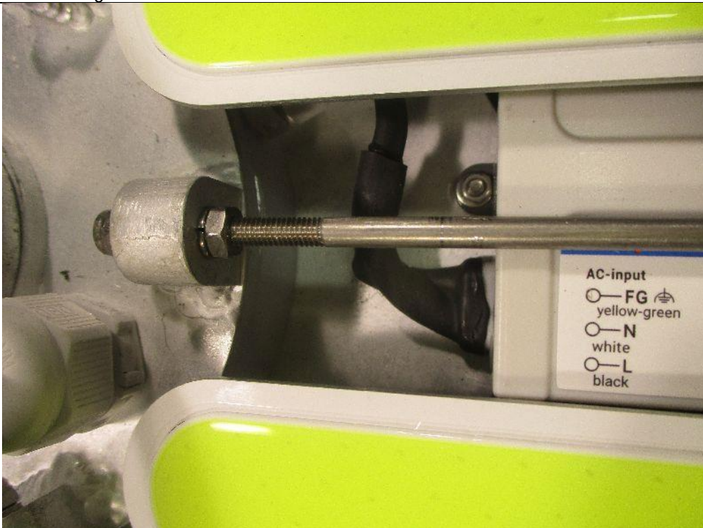
Bild / Picture 8: Securing of LED converter
